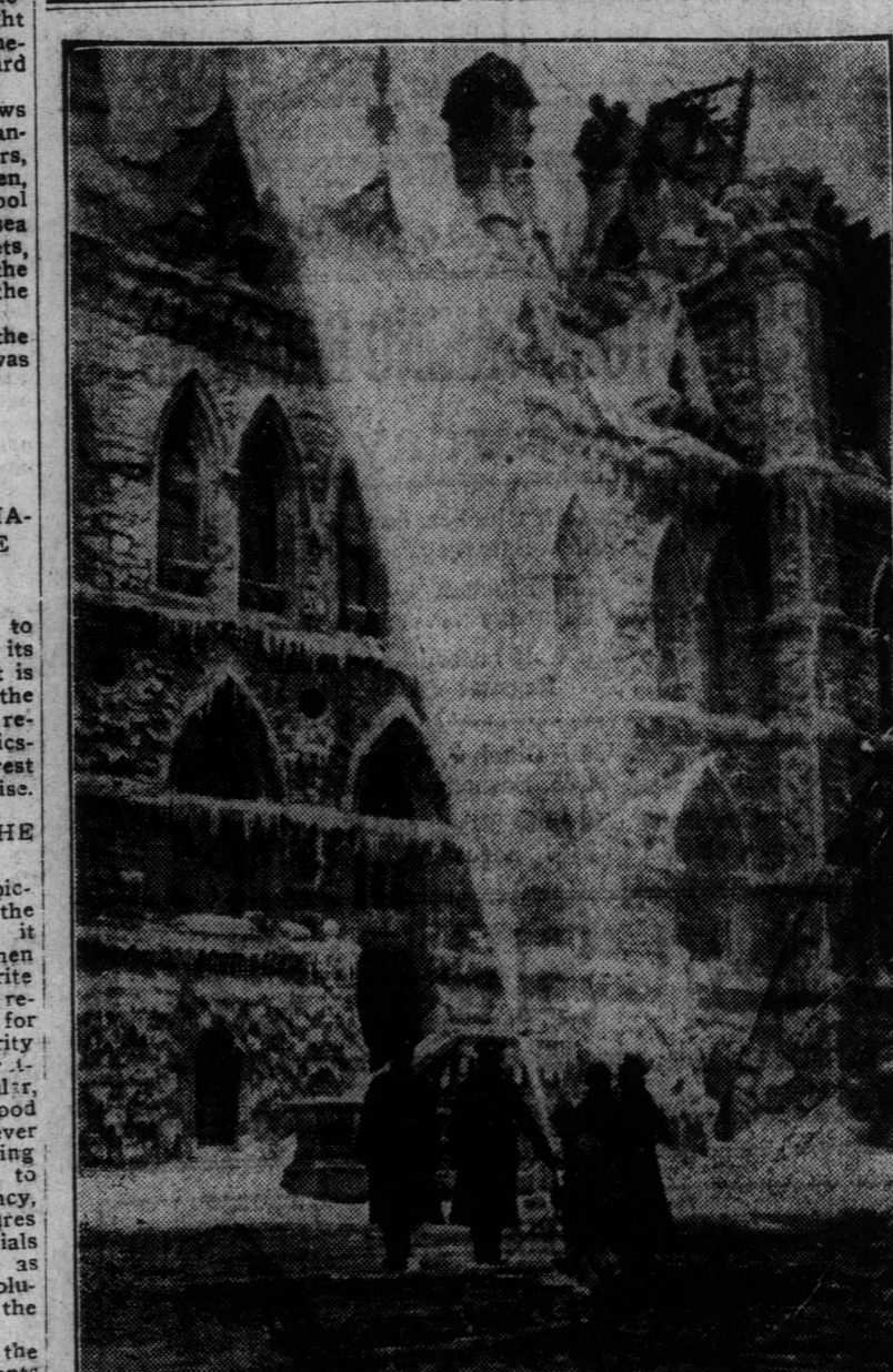
Scenes at the burning of the Parliament Buildings, which will be shown at the Apollo shortly.
