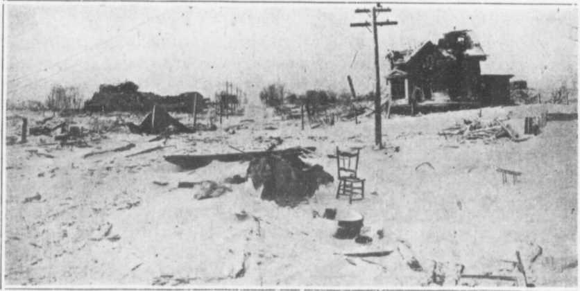
Roome Street.—School on left.
