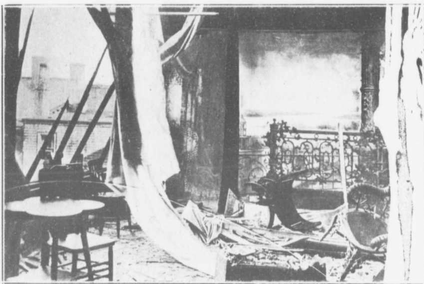
Cox Bros.' Studio.—Showing destruction wrought by explosion.
