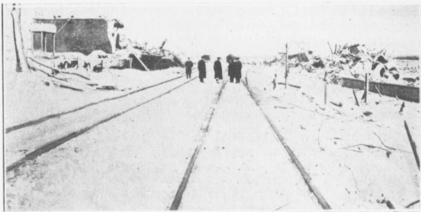
Ruins of old Acadia Sugar Refinery on right.
