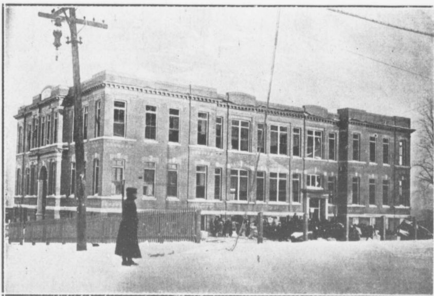
Alexander McKaye School.—Though badly damaged, it was used as a relief depot, where food was supplied to sufferers.
