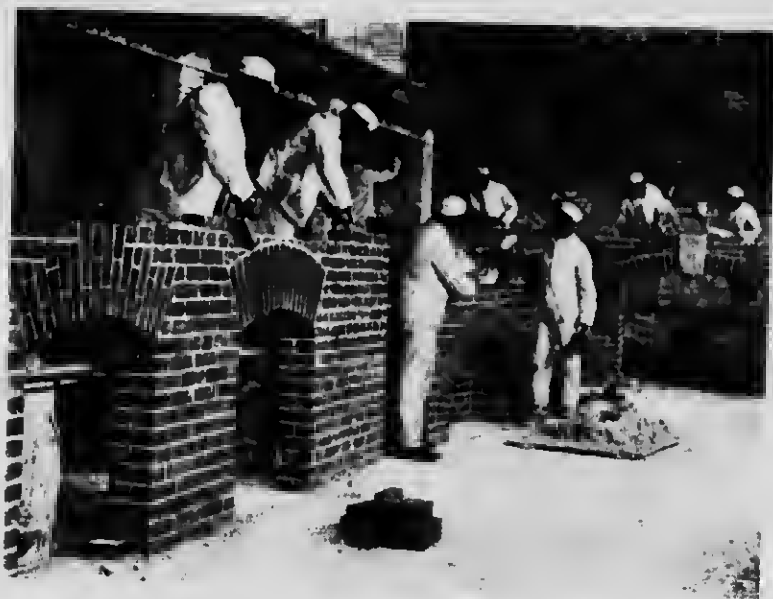
BRICKLAYING AT HAMPTON INSTITUTE
