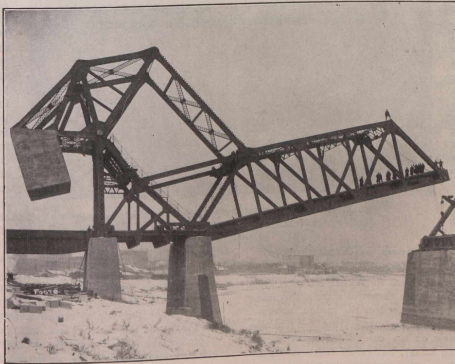
Fig. 6.—General View of Bascule.
