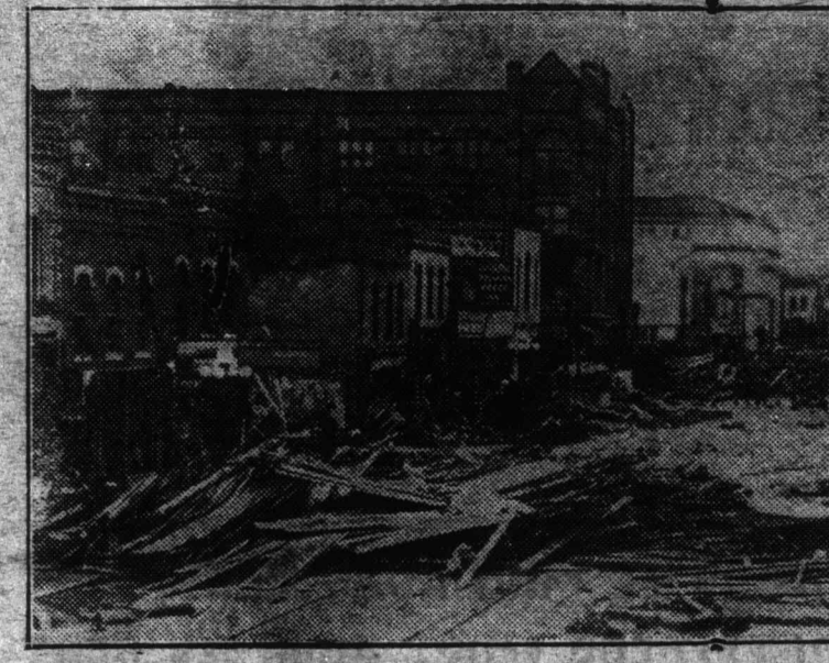
A picture taken immediately after the flood showing Union Avenue, one of the main streets of Pueblo. Note the debris on the road.
