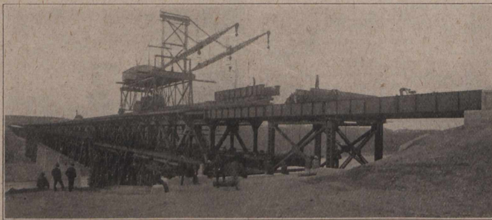
Edmonton Bridge Construction May 27, 1913.
