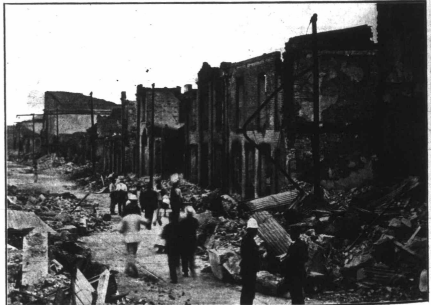
Harbour Street, Kingston, Jamaica, After the Disaster. Taken from the Treasury Steps Looking West.
