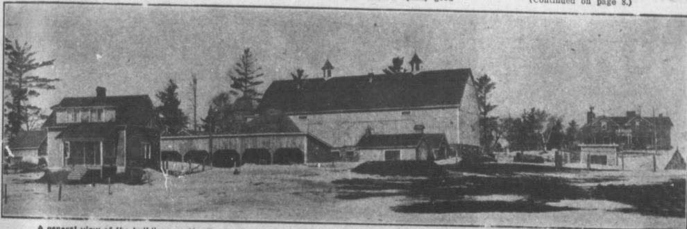
A general view of the buildings on Mr. Burnaby's farm. From left to right we have hired man's house, barns, and Mr. Burnaby's residence.
