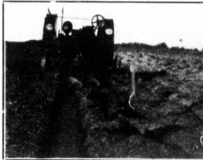
Showing the "HAPPY FARMER" Tractor pulling three 14-inch bottoms through brome grass sod 5 inches deep. Self-steering.
