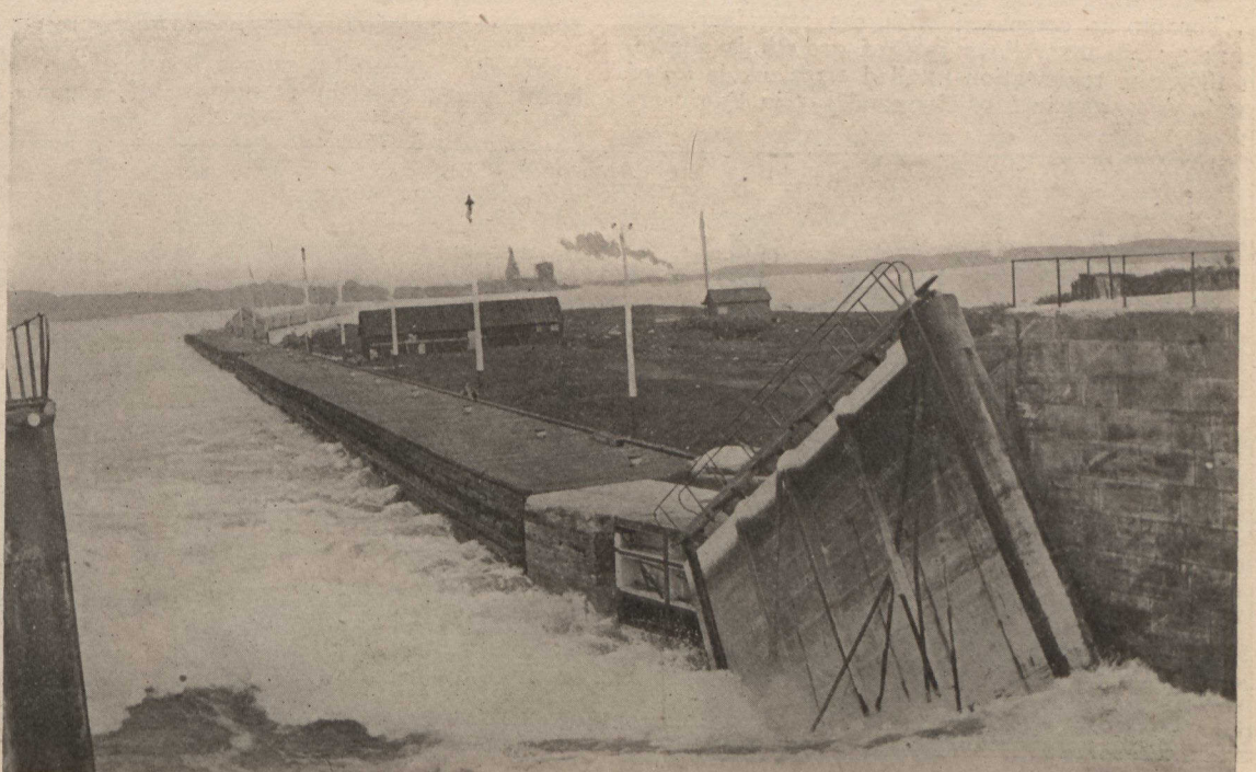
The Gates of the Sault Canal, broken last week, causing damage estimated at a quarter of a million dollars.
