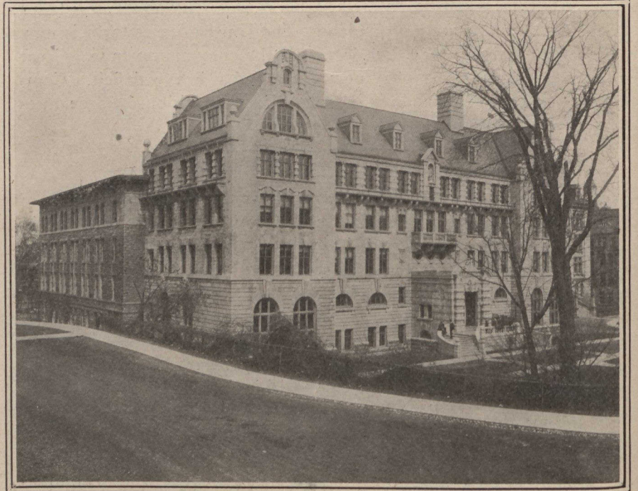
The New Macdonald Engineering Building
