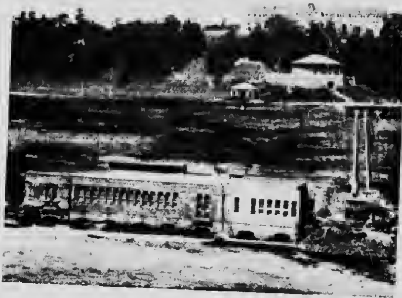
POWER-HOUSE AT NIAGARA FALLS.
