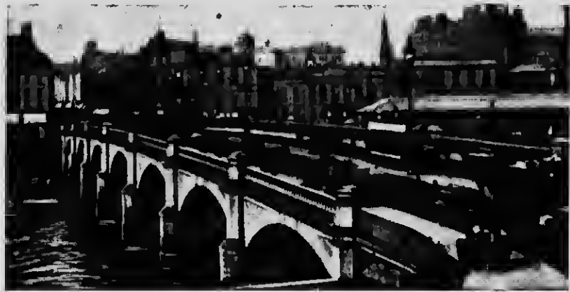
BRIDGE OVER THE CLYDE, GLASGOW.
