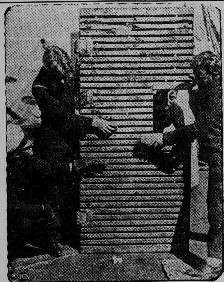
Divers off New London, Conn., have brought up the first salvage from the Navy submarine S-51, a deck grating. Under-sea workers are stripping all unnecessary weight from the boat, which sank with heavy loss of life after a collision last fall, to facilitate raising.
