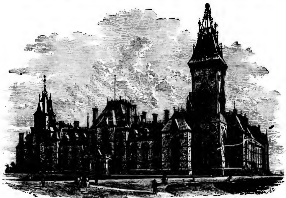
GOVERNMENT BUILDINGS, OTTAWA—EAST BLOCK.
