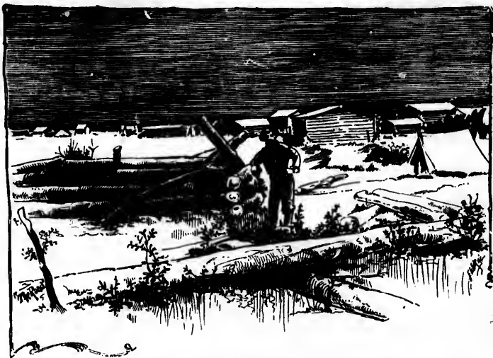
A MINER BUILDING HIS CABIN AT CIRCLE CITY.
