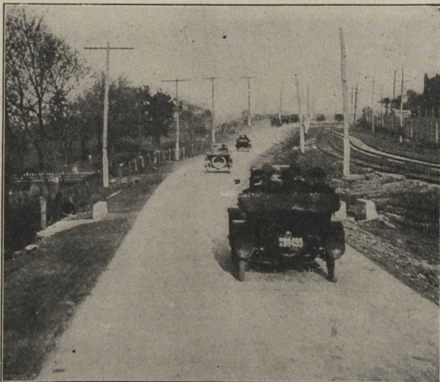
And still they come! It is a common thing these days to see an apparently endless procession of cars, on business or pleasure bound, from country to city and vice versa. The above is an illustration of actual traffic on a tempting stretch of concrete road.
