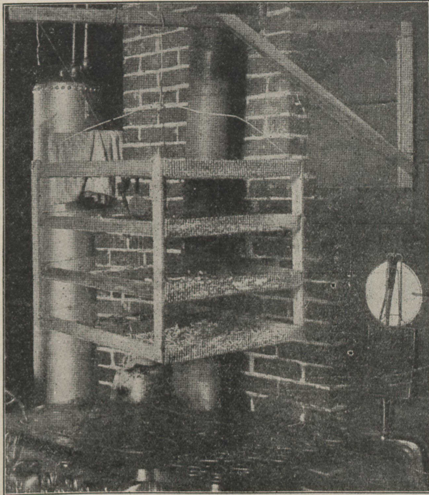
This drying-rack is hung from a wooden arm that will swing back against the wall. The trays nearest the heat will get a higher temperature than those at the top.
