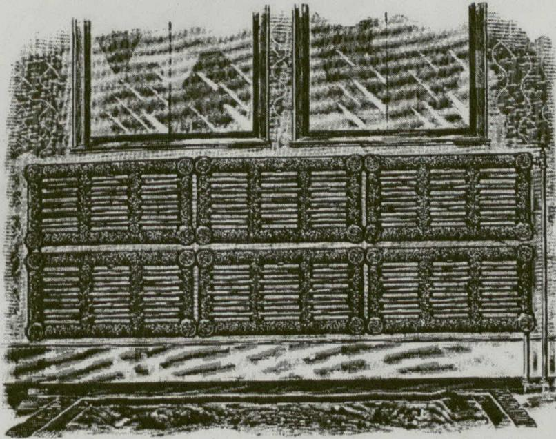
The above illustration shows a new type of Radiator suitable for all Classes of Buildings, and may be connected in various clusters of horizontal or vertical loops to fill up any required space.
