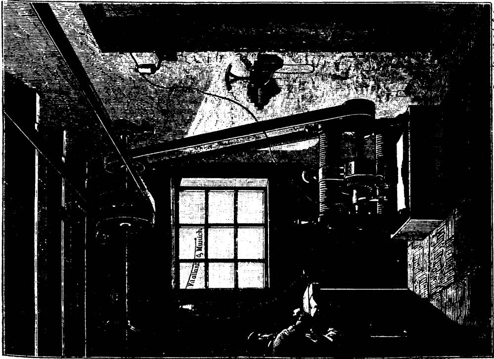
FIG. 6.—INSTALLATION AT MIESBACH.
