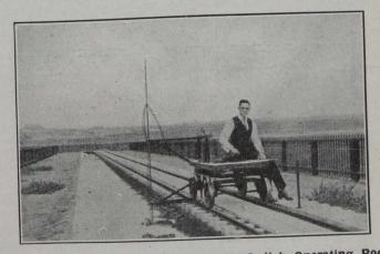
Meter Rating Car at Rest; Note the Switch Operating Rod Upright at Right and the "Time" Push Switch Opposite, near the Left Wheel.
