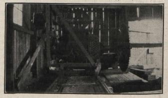
provide a bearing nearer the saw. The motor speed may be varied from 1,125 to 1,800 R.P.M. to provide for various classes of work, with saws of different diameters. This motor is rated at 10 horse-power.
