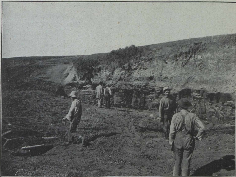
Castor, Alberta—Uncovering 7 foot Seam by Team and Scraper
