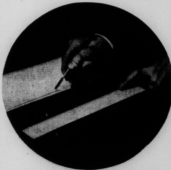
How to draw a straight line with brush and ruler.—See article.
