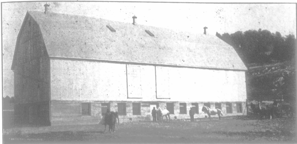
Metal Barn on Farm of J. H. Parker, Sherbrooke Co., Quebec. Note the proportion of glass to wall space in stable, insuring ample sunlight.
