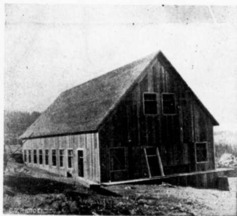
New Air Compressor Building.
