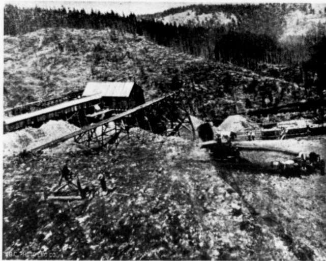
Bird's Eye View of Stripping Operations.
