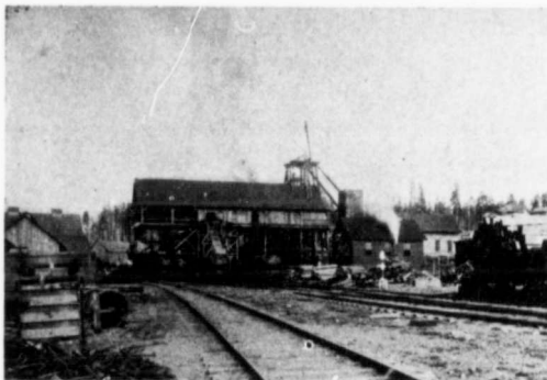
Shaft House, Knob Hill Mine.
