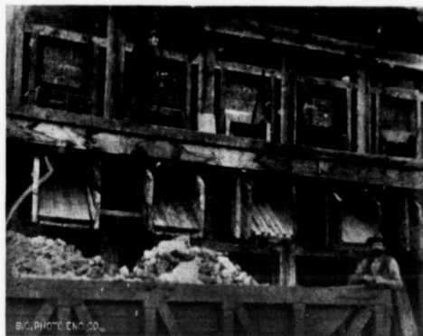
Loading Ore from Bins.
