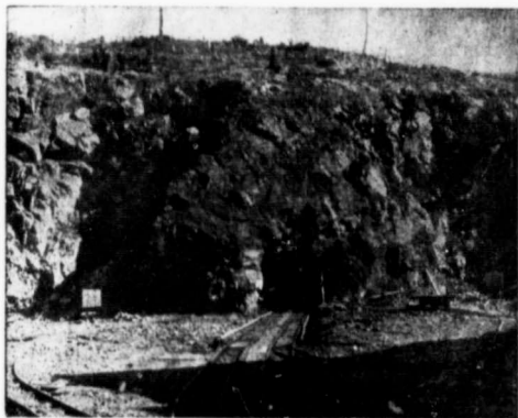
No. 3 Pit and entrance to No. 1 Tunnel.
