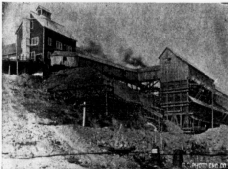
Shaft House No. 2 and Bins.
