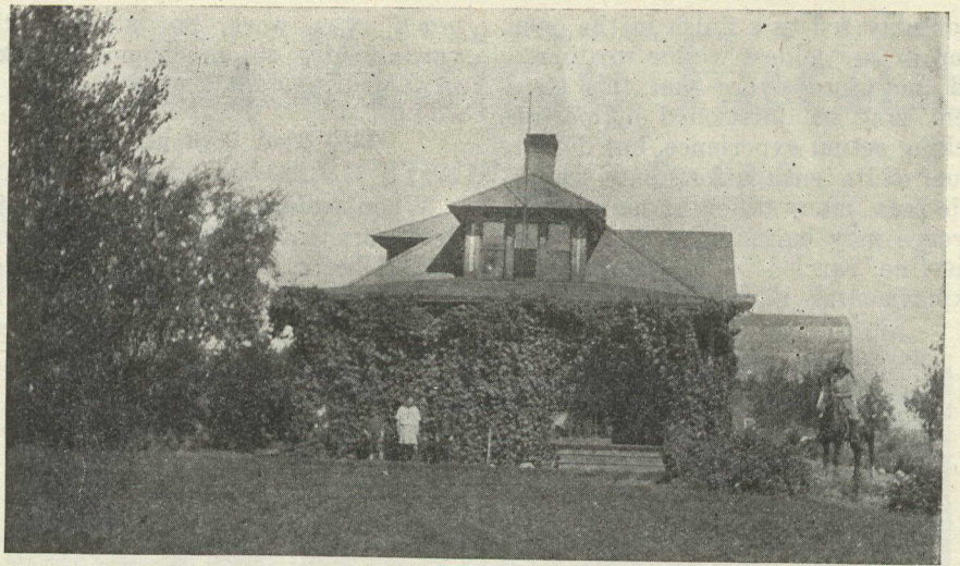
There's nothing "bleak" about this prairie home. Mr. H. A. Suggitt of Coaldale, Alberta, is a great "practitioner" of treeplanting, witness these two scenes from his farm property.
