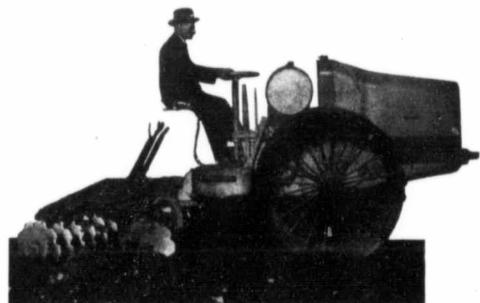
Fig. 205. Side View of the Two Wheel Two Driver Tractor built by the Providence Engineering Works.
