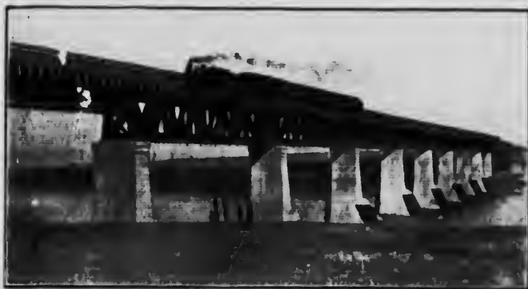
Canadian Pacific Railway Bridge—one of our five bridges.
