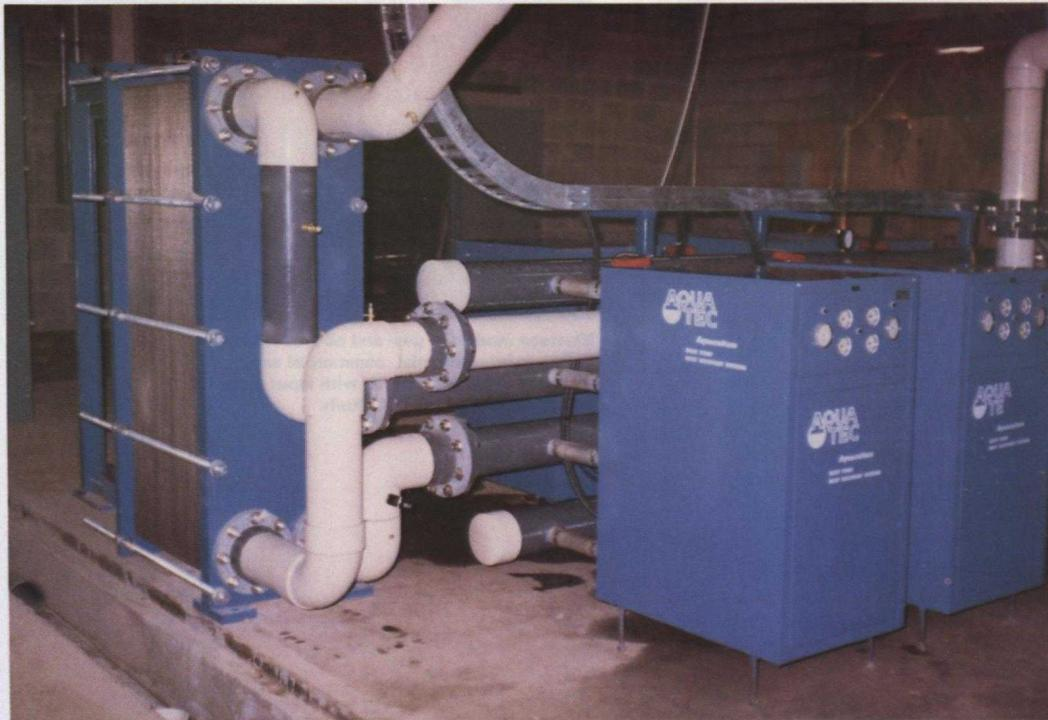
stainless steel evaporator and condenser capable of high flow (50 to 5 000 gpm) and high-efficiency ratios of 20:1 or better.
