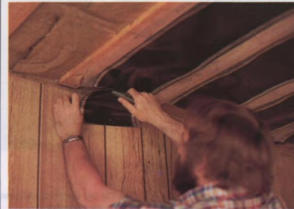
The Thermofilm electric panel heating elements.
