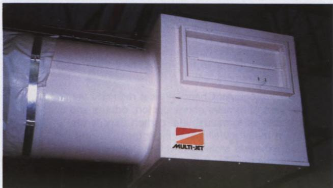
The three-in-one Multi-Jet System provides make-up air, evaporative cooling and heat recovery.
