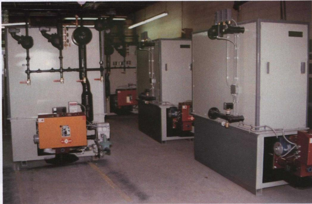
The photo shows a 6 million Btu high-pressure steam boiler on the left and two hot water boilers of 2.5 million Btu capacity each, on the right side.
