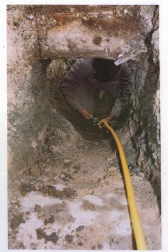
Kitec flexible pressure pipe being installed for water service distribution.
