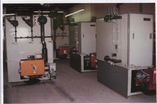
The photo shows a 6 million Btu highpressure steam boiler on the left and two hot water boilers of 2.5 million Btu capacity each, on the right side.
