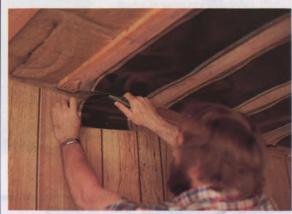
The Thermofilm electric panel heating elements.
