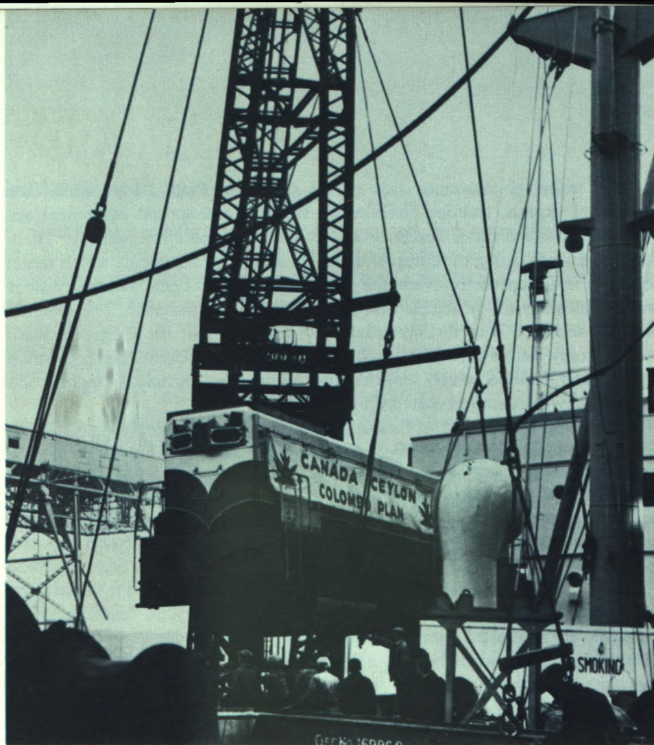
A floating crane loads a locomotive destined for Ceylon as part of Canada's contribution to the Colombo Plan.
