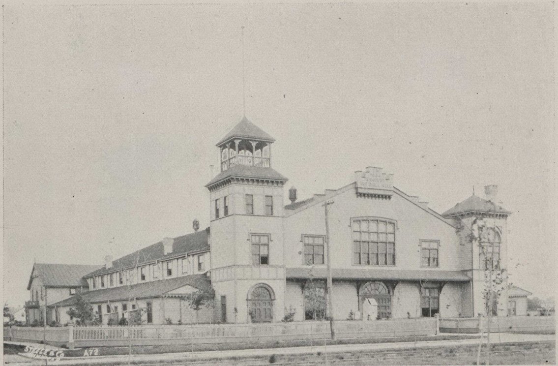
ARMOURY AND DRILL HALL—WINNIPEG
