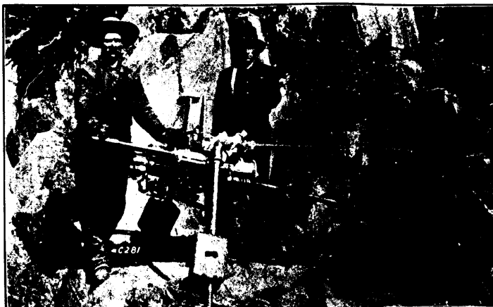
The "Little Giant" on G. T. P. Excavation Work
