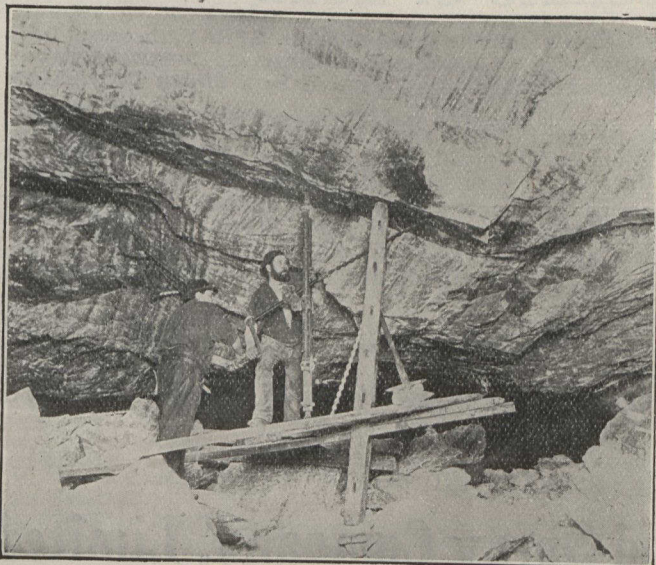
Drilling for Blasting
