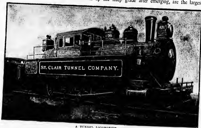
A TUNNEL LOCOMOTIVE.
