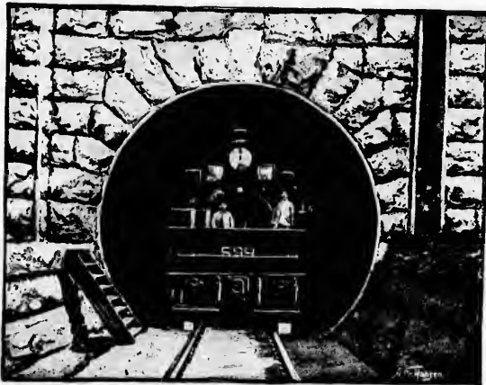
TUNNEL ENGINE EMERGING FROM PORTAL.
