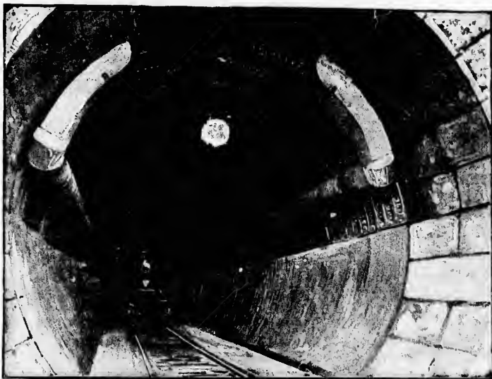
VENTILATING DEVICE, FOR REMOVING SMOKE.
