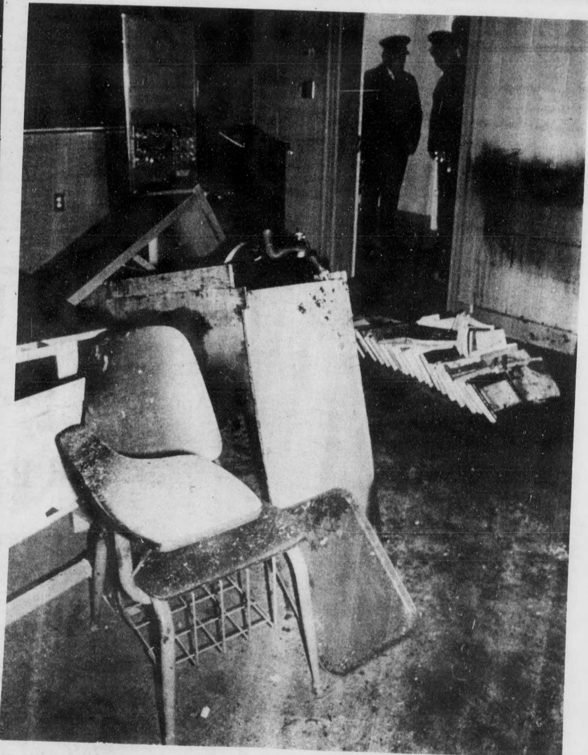
A partial view of damages to the Kierstead Hall Lounge after Wednesday night's fire. Most damage was done to the bookcase that was originally on the wall at right.
