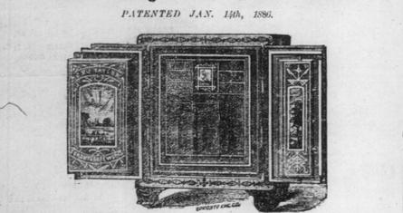
All our new Fire-Proof Safes are fitted with this latest improvement. They have also DRY AIR CHAMBER to prevent dampness. Lock protected by CHILLED STEEL PLATE to prevent drilling. J. & J. TAYLOR, Toronto Safe Works. June 27, 1887.
