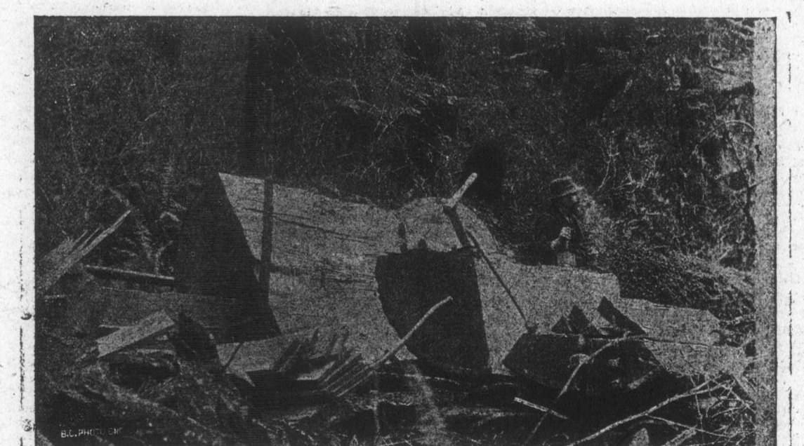
SPECIMEN SPRUCE, QUATRSINO.—This is how the settler gets material for building his house. The spruce will split into boards feet long, as fine as if sawn.
