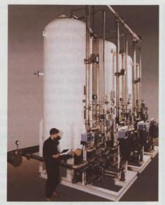
Glegg Water Conditioning, Inc. Mixed Bed Polishing Units.
