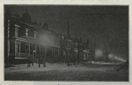
The streets of Outremont are well-lighted at night. Over 500 electric arc lamps of the latest pattern being recently installed
