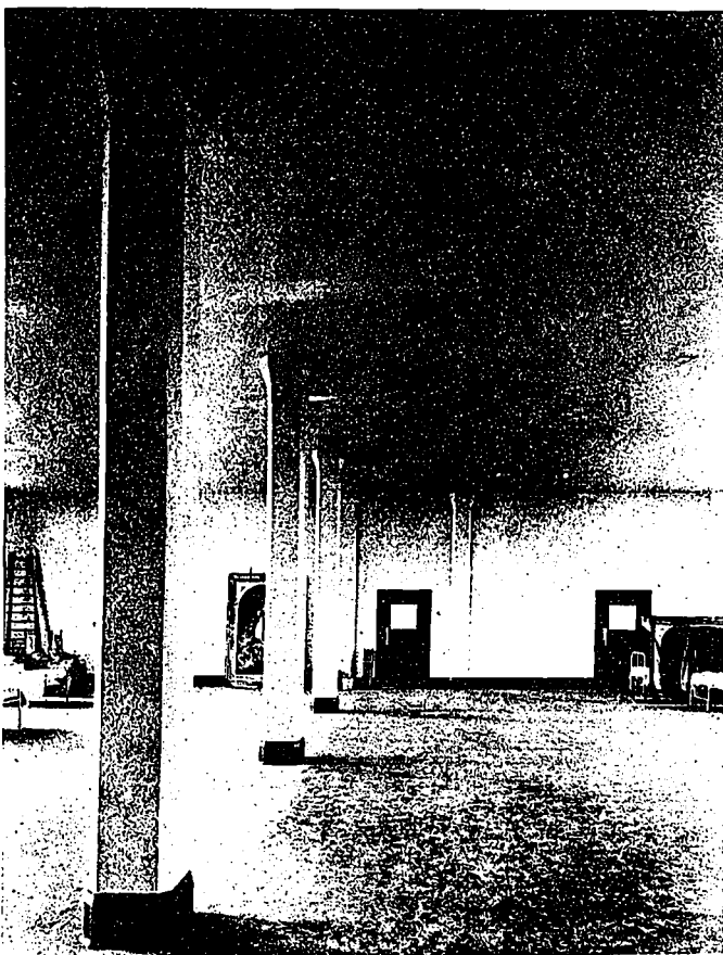
REINFORCED CONCRETE COLUMNS IN DORMITORY, DE LA SALLE TRAINING COLLEGE, OAK RIDGES, ONT.
