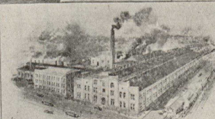
NEW FACTORY BUILT IN 1895 SINCE THEN THE FOLLOWING EXTENSIONS HAVE BEEN MADE MACHINE SHOP LENGTHENED 140' NOW 440 x 120 BOILER SHOP 100' NOW 220 x 50 WITH CORRESPONDING INCREASE MOLDING SHOP 100' NOW 150 x 50 IN EQUIPMENT. BLACKSMITH SHOP 40' NOW 100 x 40
