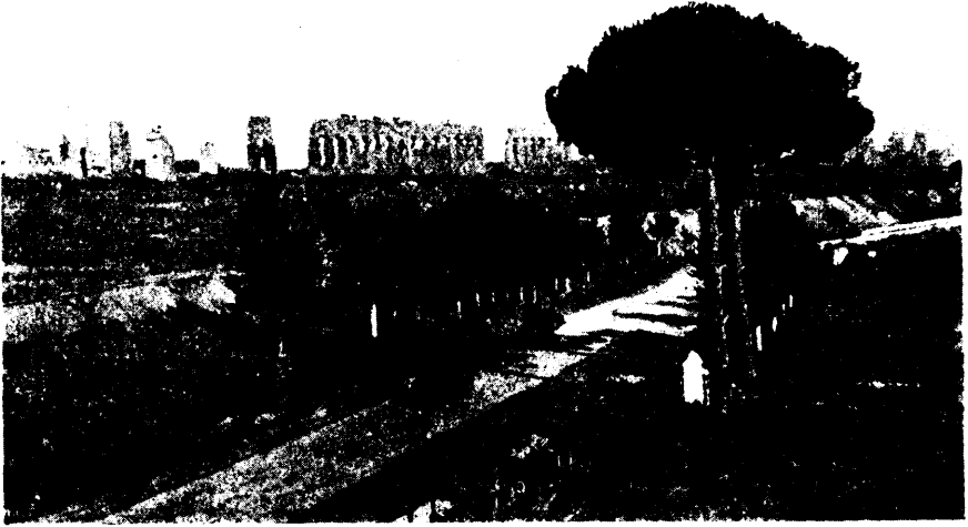
RUINS OF THE CLAUDIAN ACQUEDUCT, ROME.
