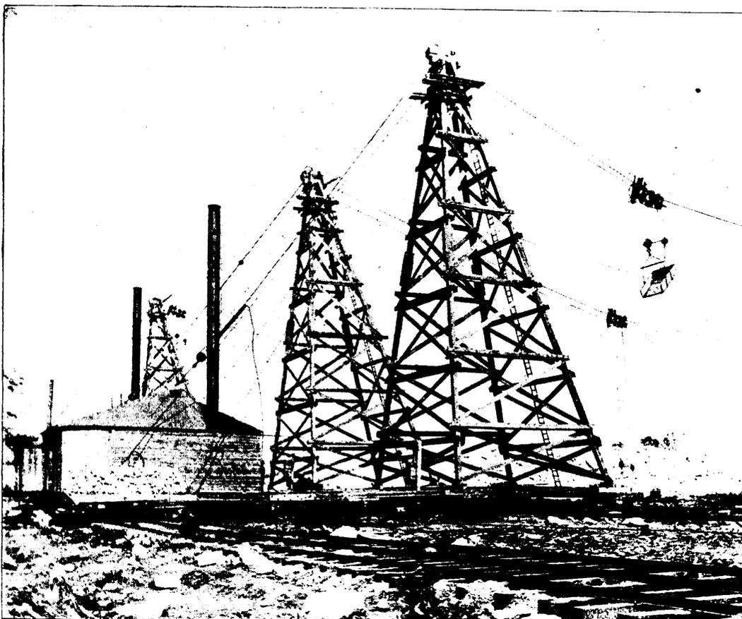
FIG. 8.—Head Towers, Traveling Cableways.
