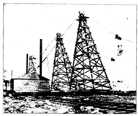
Fig. 8.—Head Towers, Traveling Cableways.
