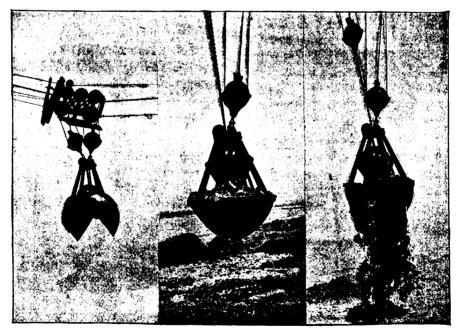
Fig. 9.—Self-filling Grab Buckets at different stages.
