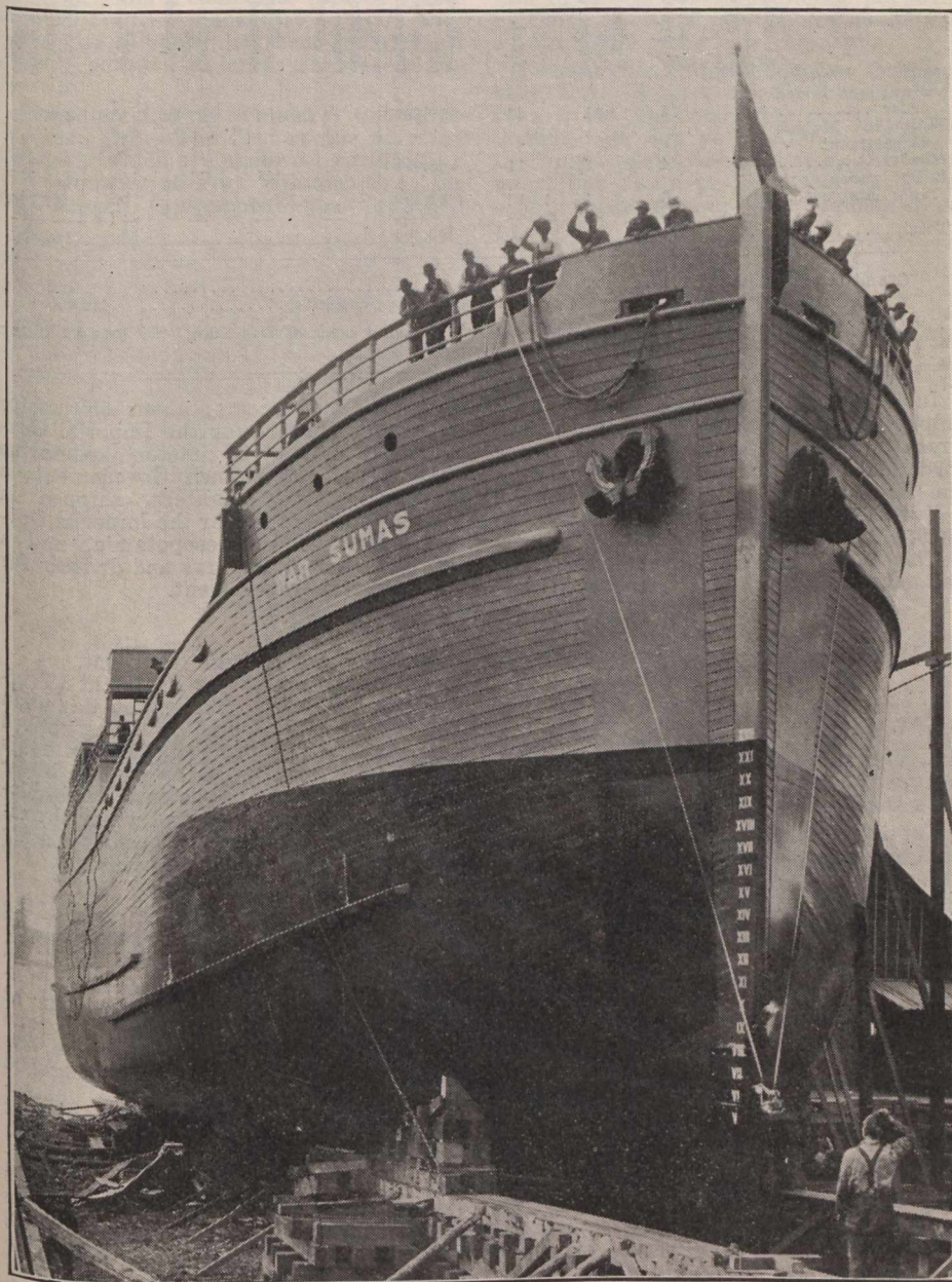
Wooden cargo steamship, War Sumas, for British Government, just prior to launching by Pacific Construction Co., at Port Coquitlam, B.C.
