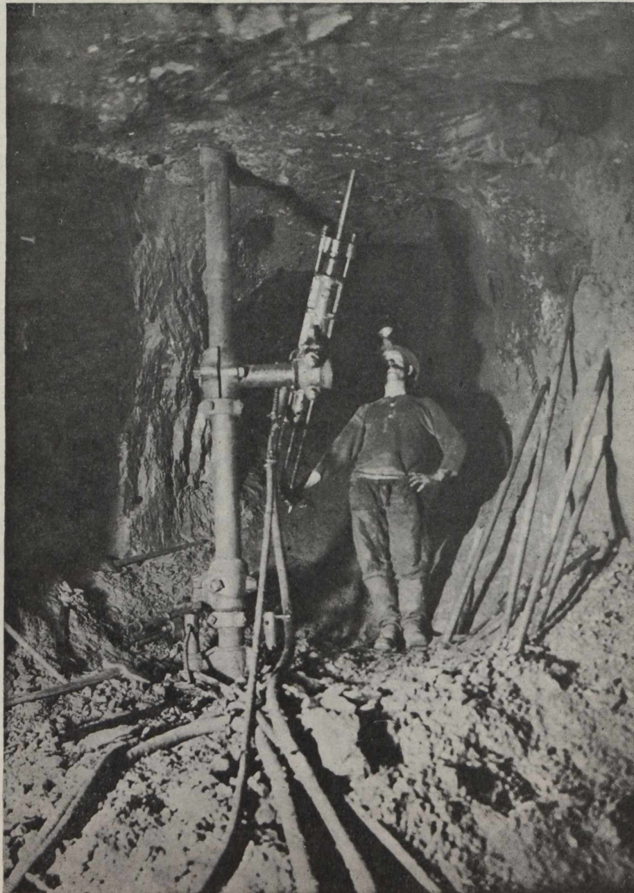
One-man (Leyner) drill, 59th level, Conglomerate lode. Calumet and Hecla mine, Calumet, Mich.
