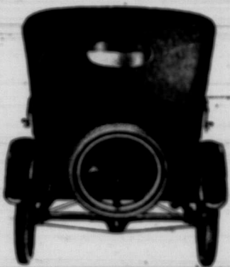
Rear View showing extra tire, tire carrier, and tail lamp with license bracket attachment.
