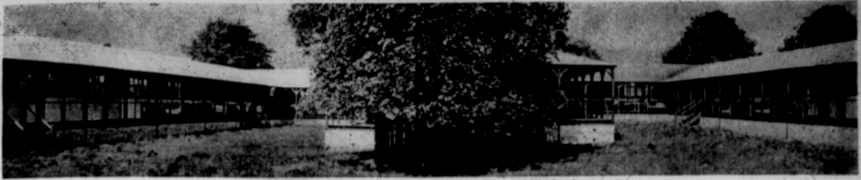
The King's Canadian Red Cross Convalescent Hospital, Bushey Park, showing the Hut Wards
