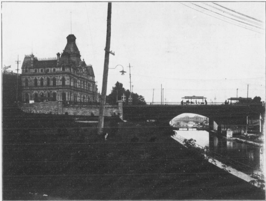
POST OFFICE AND VIEW ABOUT SAPPER'S BRIDGE
