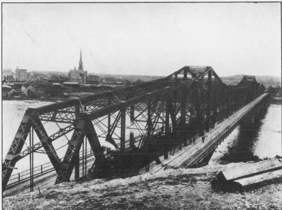
TESTING THE INTERPROVINCIAL BRIDGE
