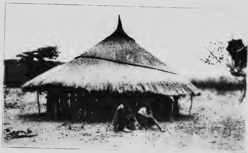
HUT OF THE UNGRIMI. THE ROPES THAT HOLD THE THATCH ARE TWISTED OF GRASS
