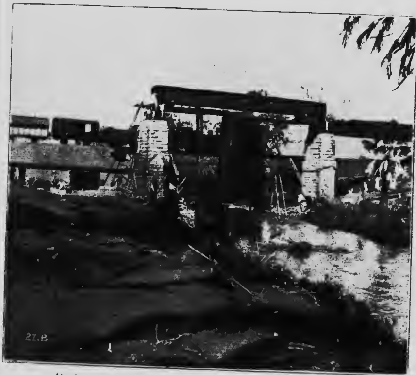
"AND FINALLY LOWERED GENTLY INTO POSITION."
