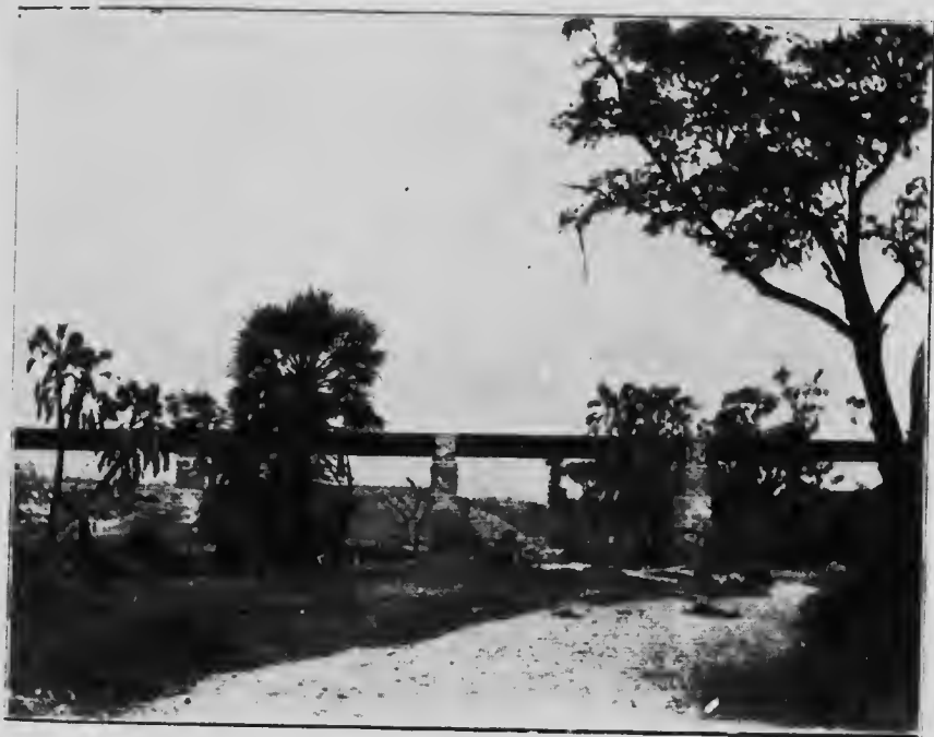
THE COMPLETED TSAVO BRIDGE.
