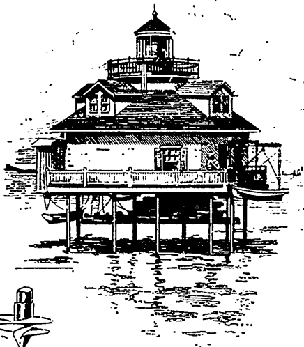
SCREW AT END OF PILE. | SCREW-PILE RIVER LIGHTHOUSE.
